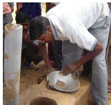
A demonstration on making smokeless chulhas (fuel-efficient cooking areas) for young people from Munda Tribe (Longa village, Khunti district, Jharkhand State)
