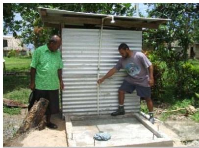
A new water supply system being installed in Natuva village, December 2008
